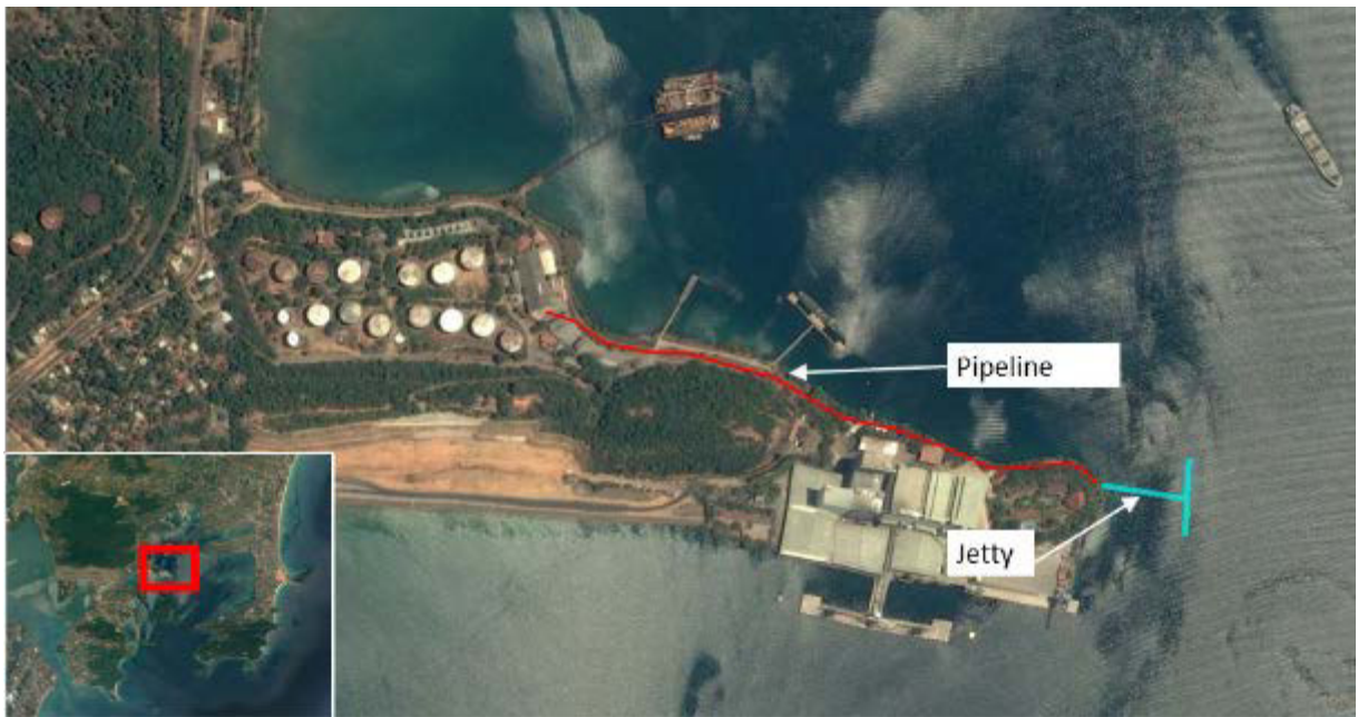
Figure 1-23: Deep-water Oil Jetty
